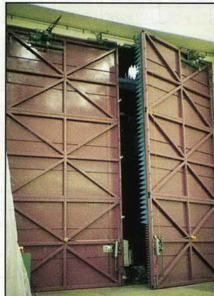
Lockheed Electric Door Operators and Pneumatic Cremona Bolts (36'x36' opening)
