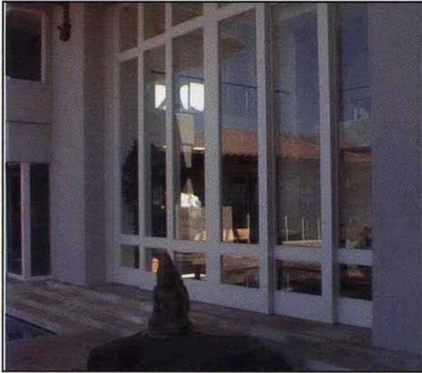
Electrically Operated #1265 Operator Bi-Parting Telescoping Wood Framed, Glass Doors (18' Tall) Maui, HI Residence
